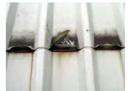
Leathergrain alternative on hot dip galvanised steel substrate roof after 7 years.
